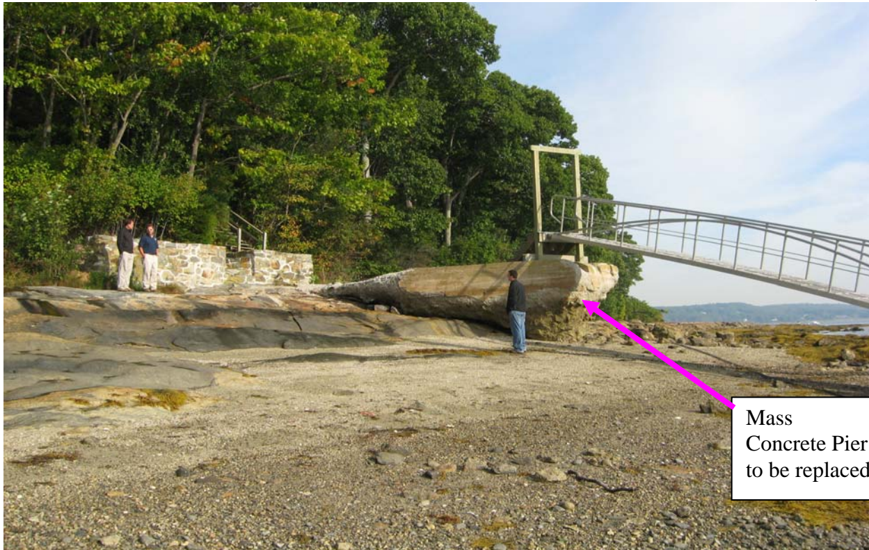
View of existing mass concrete structure that is deteriorated and requires replacement.
