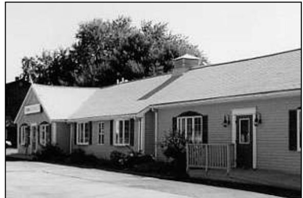
Façade step-backs and a cupola reduce the scale, trim work and window types fit local character.
