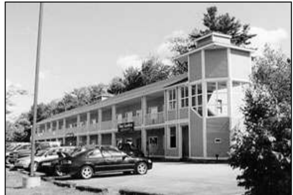
Focal points such as the tower add visual interest and help reduce the apparent scale of larger structures.
