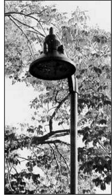
A close-up of the "bell" fixture shows its recessed lighting element and flat lens – light trespass is eliminated.
