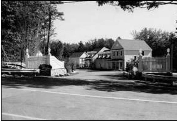
Example of a well-designed curb cut: it is no wider than it has to be, the fencing makes its location clearly discernable to the motorist, and it is attractively landscaped.
