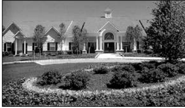
Human-scale building elements and a generous landscape treatment create a desirable living environment.
