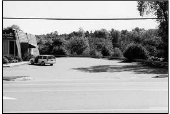
Example of a poorly designed curb cut: it is far too wide for its purpose, there are no clear cues to the motorist as to its location; and it lacks landscaping all together.
