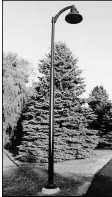
This architecturally designed "bell" fixture is attractive and functional, shedding light only downward.
