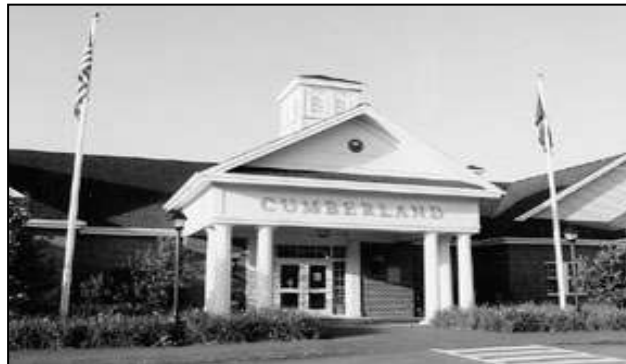
The main entrance to this building is indicative to changes in materials and roof lines, and the introduction of columns.
